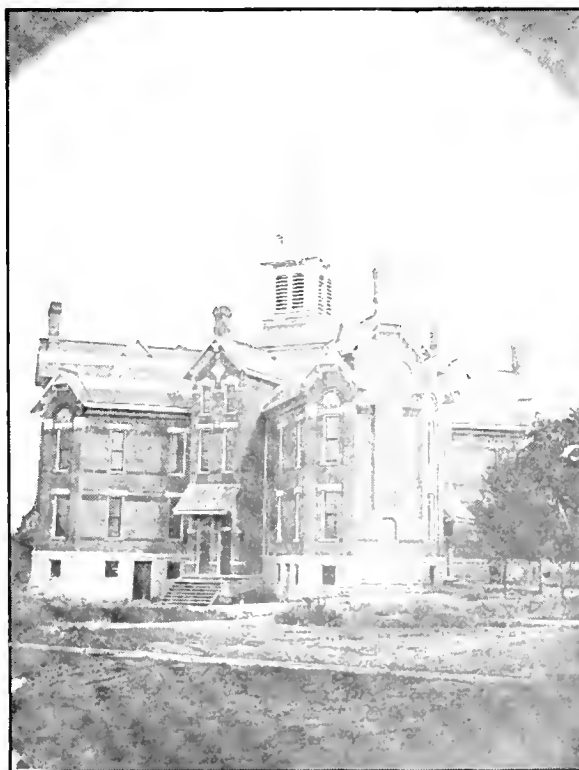
VANDALIA HIGH SCHOOL BUILDING.
